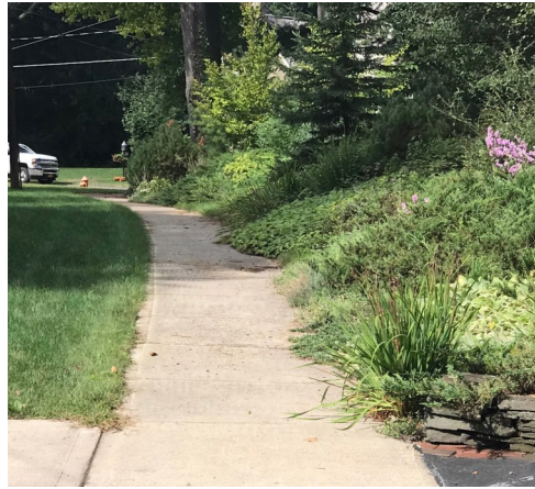
Overgrown vegetation along right edge of sidewalk
