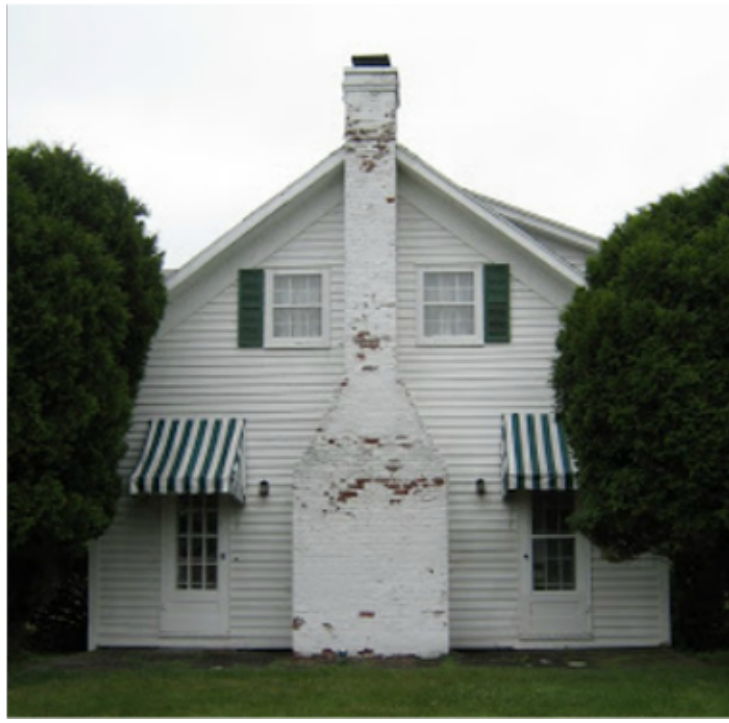
Two doors used by generations of children - one for boys and one for girls - recall the original use of 1001 Hanshaw Road in Cayuga Heights
