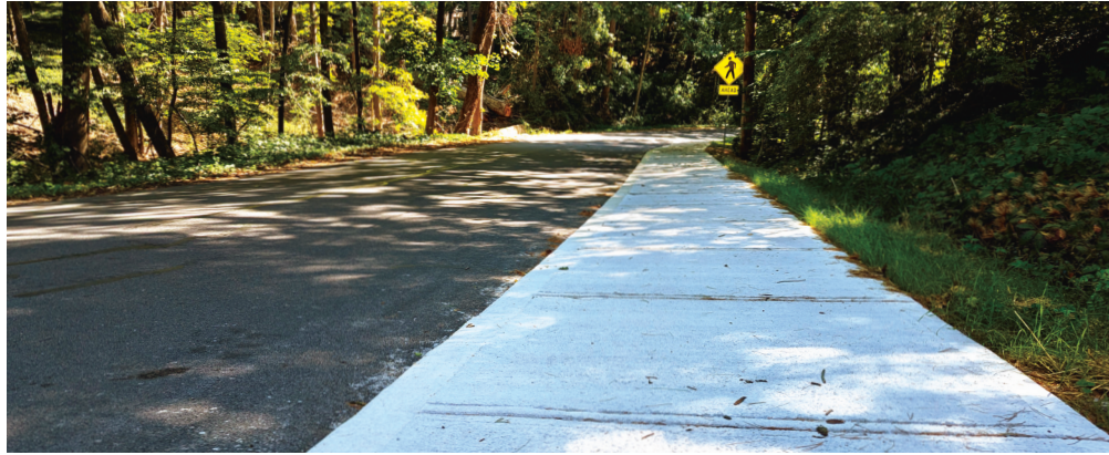
Wyckoff Road sidewalk - built by our own DPW
